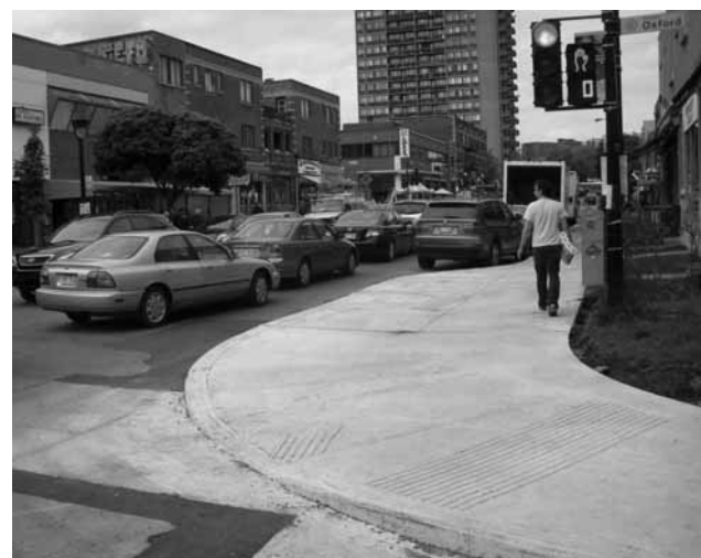
Large, round concrete eyesores were built on many Monkland Ave. street corners, taking up parking spots and enraging merchants.
